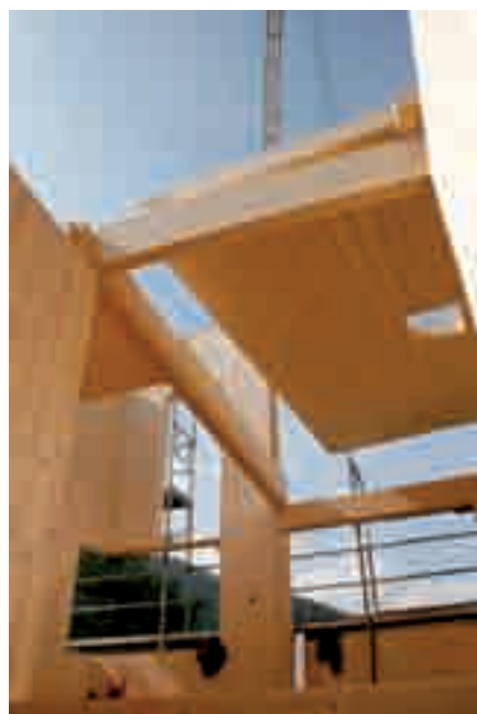
Montage Massivholzelemente © Holzius
