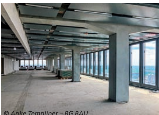
© Anke Templiner – BG BAU
