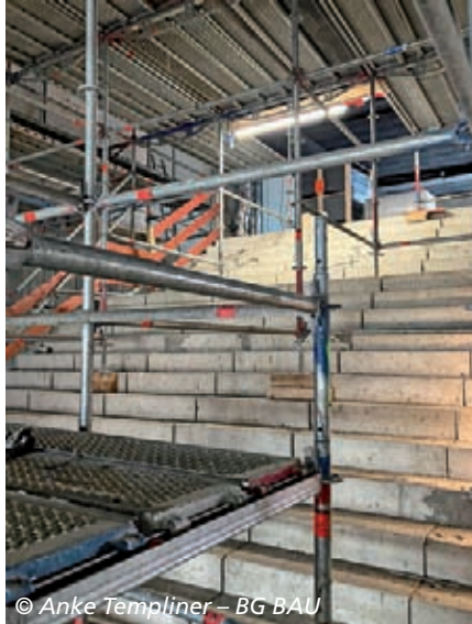
© Anke Templiner – BG BAU
